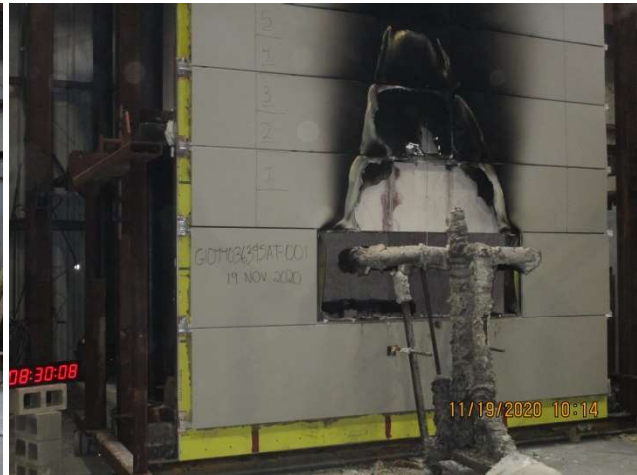
Completion of Phase 2 NFPA 285 Test
